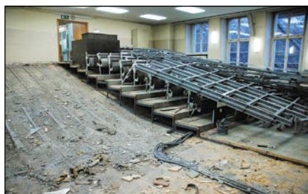
Abriss des alten Hörsaals (Dezember 2004) Demolition of the old lecture hall (December 2004)
